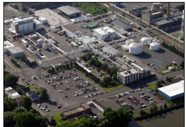
Industrial land uses such as Organichem are valuable economic assets, and should be encourage to continue to operate in Rensselaer.
