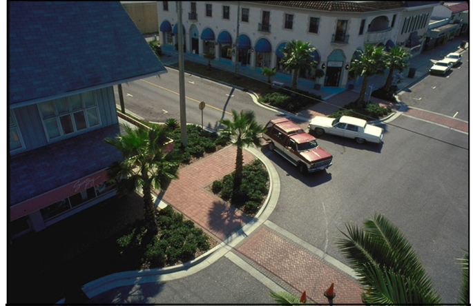
Textured crosswalks and sidewalk bump-outs at intersections calm traffic and create a safe pedestrian environment.
